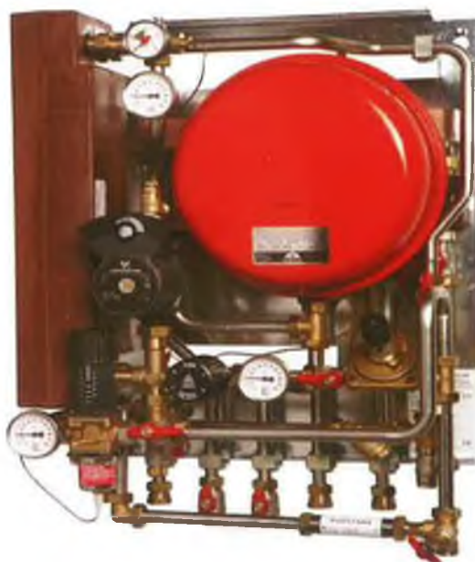
Figure 20 - indirect plate heat exchanger unit
